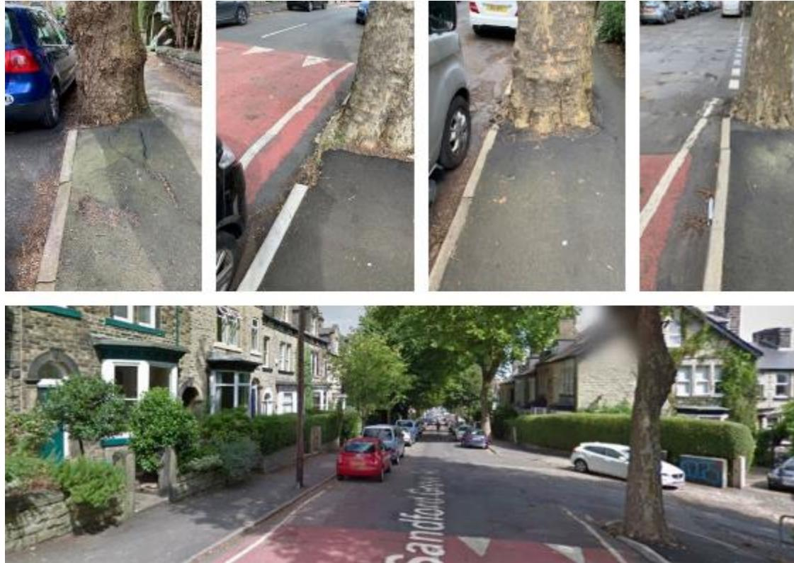
**Top right photo:** located on the junction of Marden Road, the kerbs have been displaced with an asphalt infill in place. There is no visible evidence of rooting into the carriageway. Both footway and carriageway resurfacing remain outstanding;
