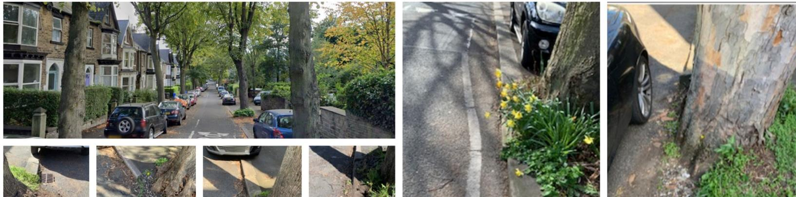
The photos above are a sample of the issues to be addressed such as missing kerbs and tree buttress roots extending into the carriageway. Out of the thirteen (13) trees of concern, up to eight (8) trees along the length of Steade Road are impacting on the kerb line, with kerbs either missing or displaced and with roots potentially extending into the carriageway. Overall, the footway defects consist of minor ramping and cracking due to tree roots.
