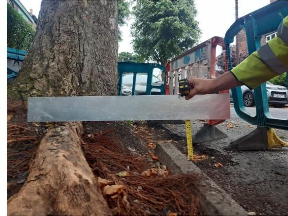
The photos above show the extent of the roots running along the footway, up to an under the private boundary wall causing damage. The upstand of the roots above the footway / kerb face is 180mm.
