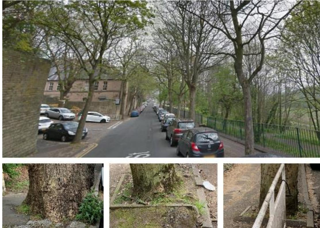
The photos above show the common defects that exist along the length of the road, from minor kerb displacement, raised tree pit edgings and footway defects that need to be addressed.
