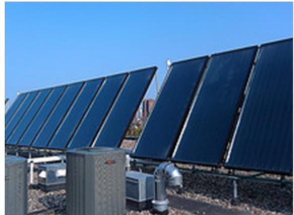
Figure 25 . Flat plate collector
