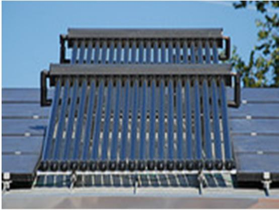
Figure 24 . Evacuated tube collector
