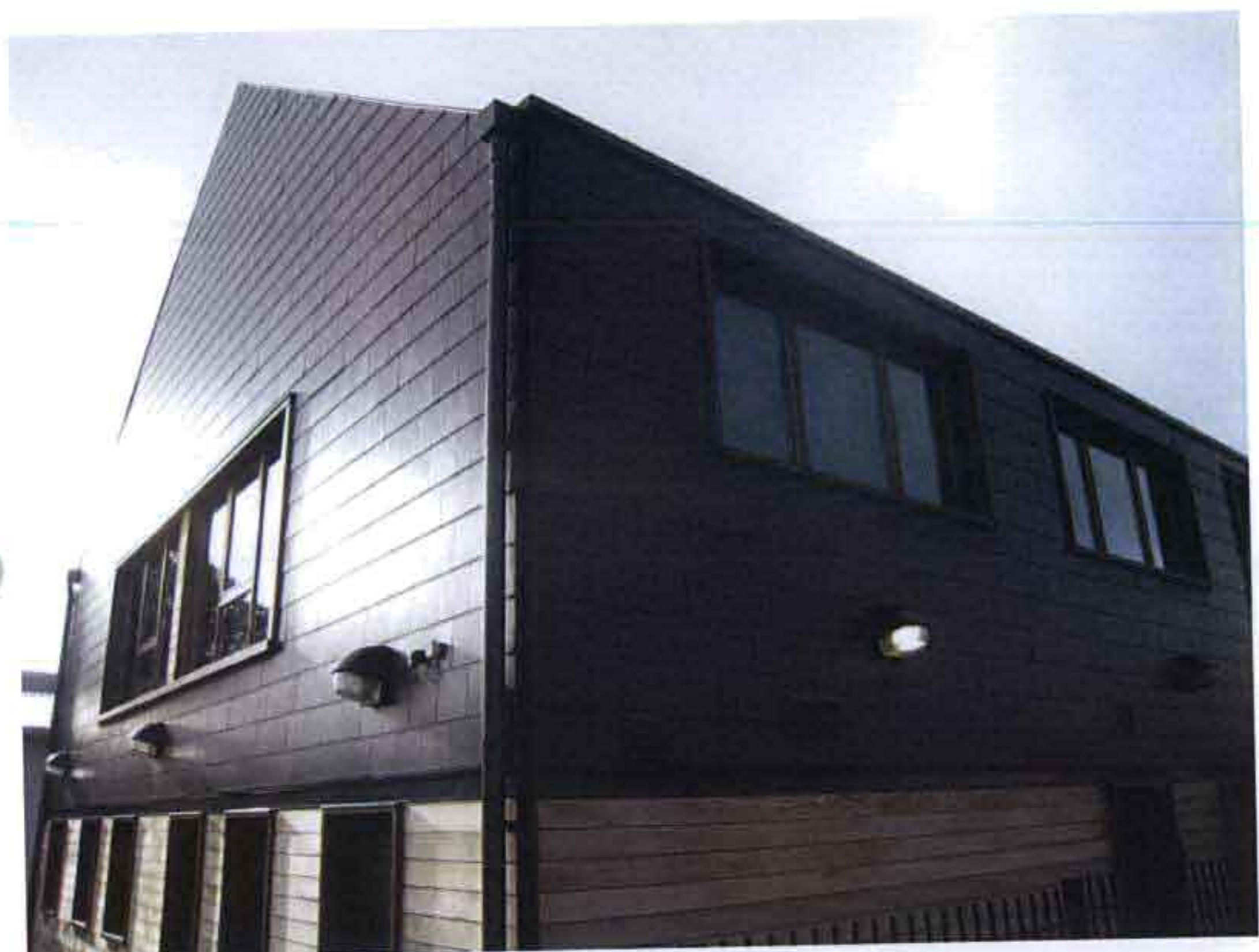
Shirecliffe Community Centre
