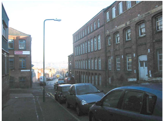
63. View north-east along Upper Allen Street - the Stephenson Blake buildings are on the right.
