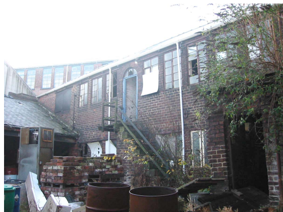
59. Courtyard to the rear of 35 Well Meadow Street (1) - note the original workshop fenestration.
