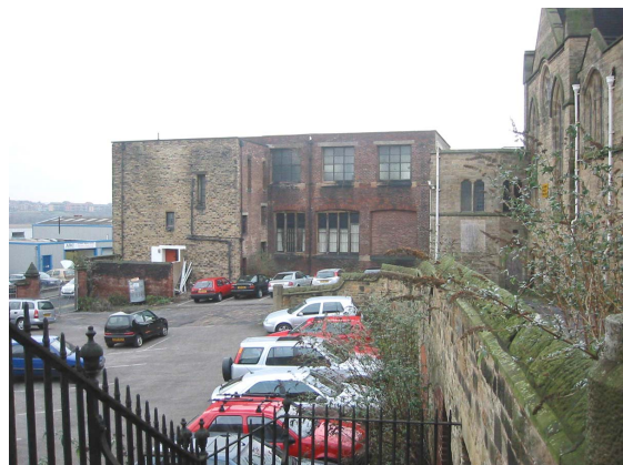
47. The grounds of the church are currently used for city-centre parking.
