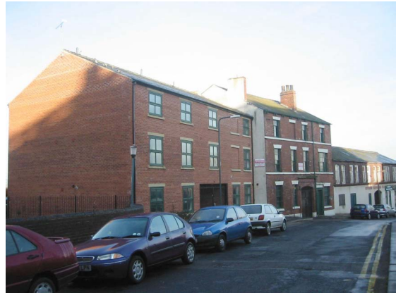
67. Looking north-east along Solly Street at the Cambridge Works (6) centre-right (listed Grade II) - to the left sits an insensitive extension.
