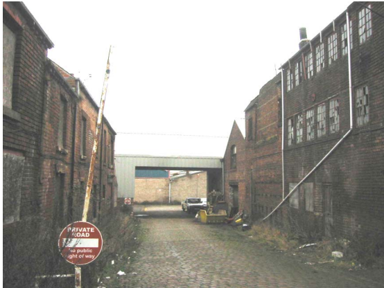
60. Looking north-east along Well Meadow Street.
