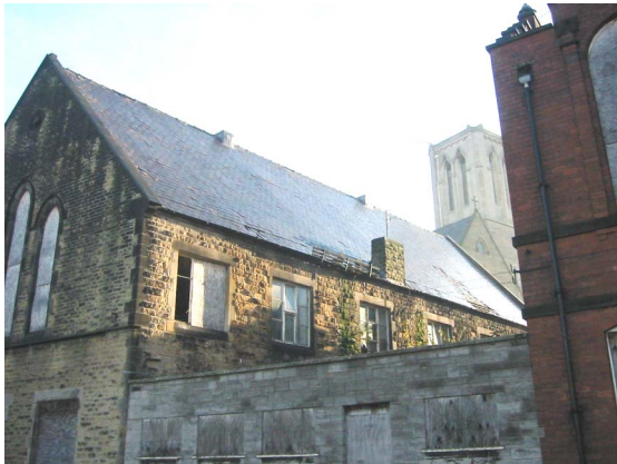
44. Church Hall building on Solly Street - currently unused.
