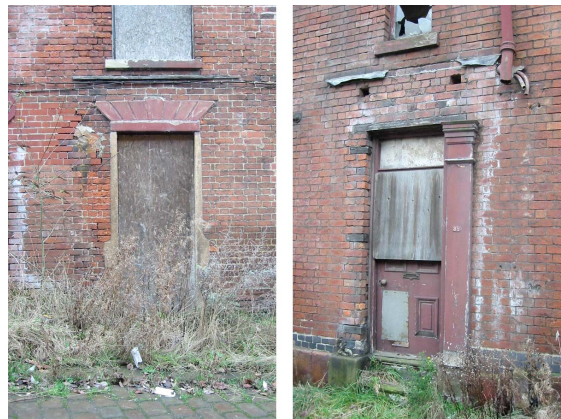
57. Entrance doorways to 35 Well Meadow Street - note the multi-keystone lintel on the example on the left.
