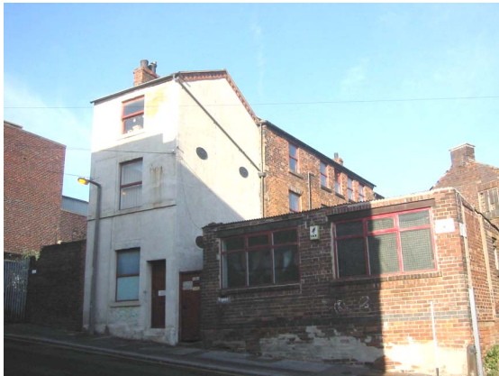
74. The Grade II listed 52-56 Garden Street (7) - early 18th century houses converted to workshops with adjoining workshops to the rear.
