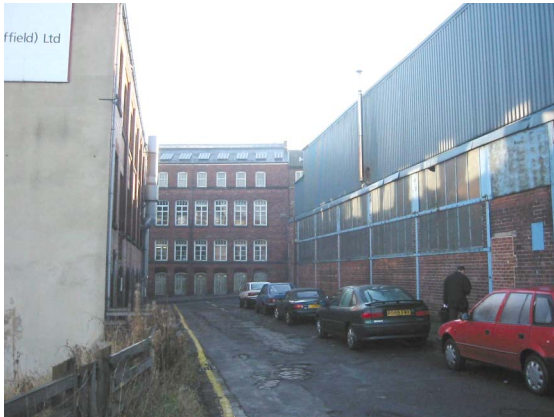
62. Looking south-east along Well Meadow Drive - the Stephenson Blake complex (4) can be seen at the end of the street.
