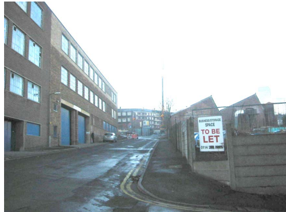
51. View looking south-west along Edward Street - in the distance are the Edward Street flats (12).
