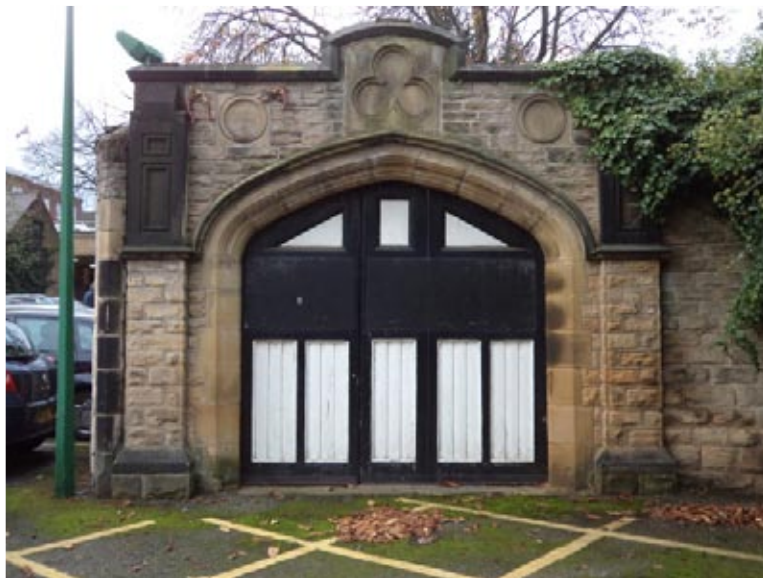
Figure 25: Outbuilding in car park
