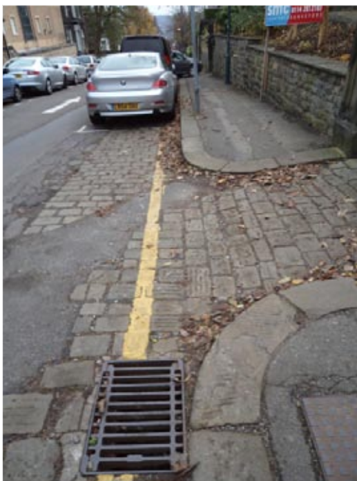
Figure 11: Stone Setts in the road
