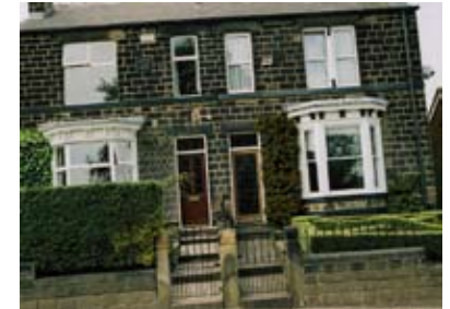
Few houses in Grenoside have retained their original doors and windows, as these houses in Norfolk Hill demonstrate; note too the burglar alarms, trailing wire and satellite dish.
