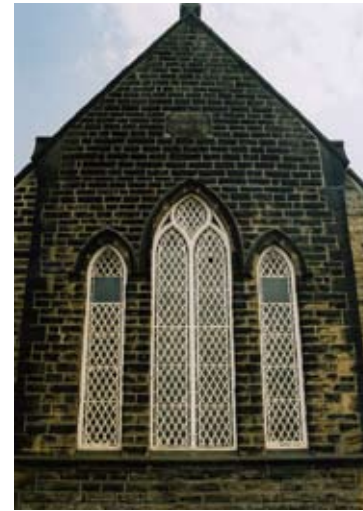
Norfolk Hill Methodist Chapel (1861) has heavy iron diaper pattern glazing to the windows.
