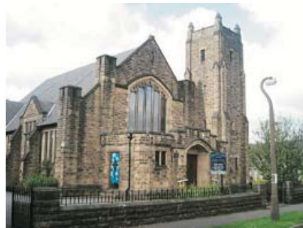
An unlisted building that makes a positive contribution to the conservation area.
