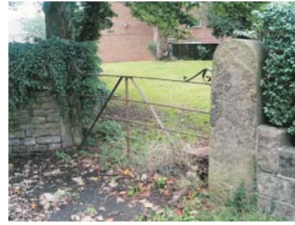
Stone gate pier and iron gate once belonging to Greenhill Hall (demolished)
