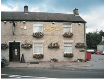
These modern windows look out of keeping with this historic building.
