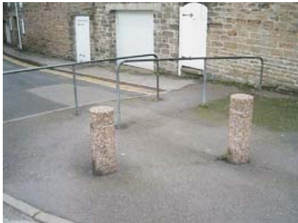
Poor quality bollards and railings spoil the setting of the adjacent listed building.
