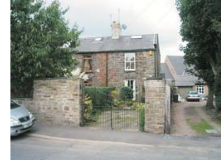
Small changes such as rooflights, satellite dish and modern windows can spoil the original appearance of a historic building
