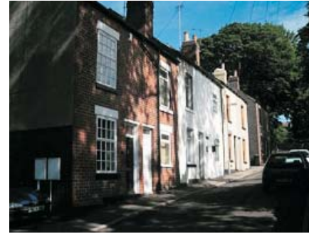
Original windows and doors have been replaced in these cottages in Chorley Road.
