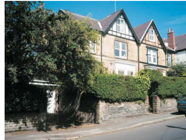
Semi-detached houses in Brookhouse Hill
