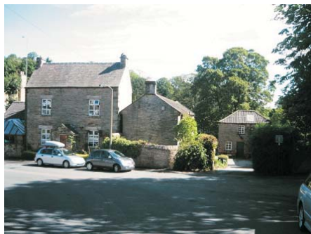
Looking east along Whiteley Lane
