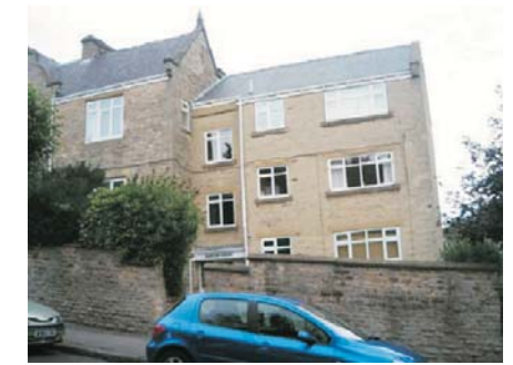
The windows in this large extension are uncharacteristic of the conservation area.
