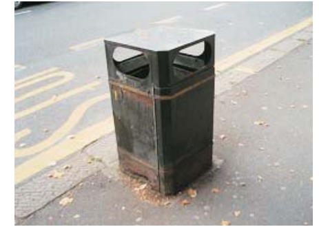
Litter bin in need of replacement.
