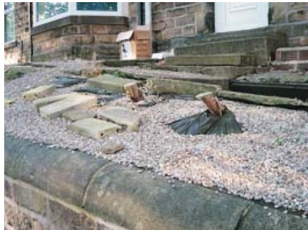
Arid area to the front of a house in multiple occupation
