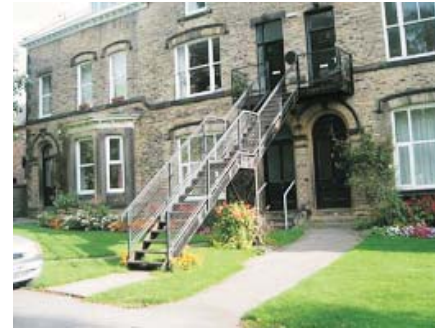
Dwelling converted to flats has resulted in these external metal stairs.
