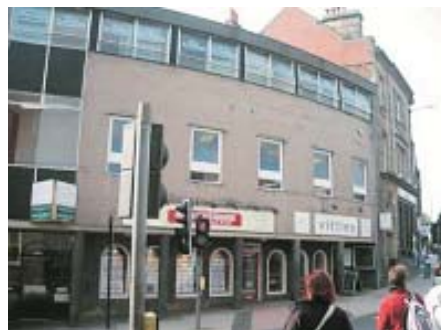
This buildings scale, proportions and use of materials (except the colour of brickwork) are completely out of character with neighbouring buildings.
