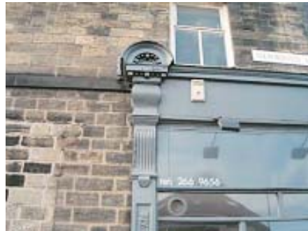
Remnant of a historic timber shopfront.
