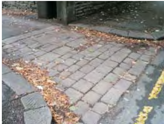
Natural stone paving along drive to No. 9 Collegiate Crescent
