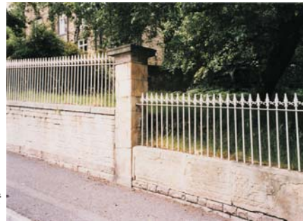
Boundary walls with original iron railings at No. 132 Upperthorpe.
