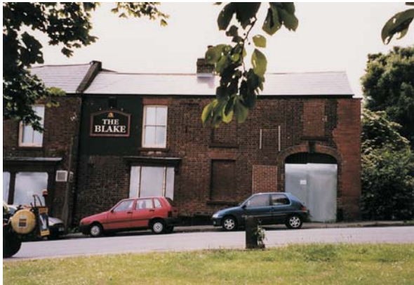
The Blake Pub backs on to the conservation area and is currently boarded up.
