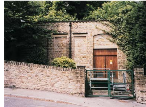
The electricity substation on the corner of Howard Road and Upperthorpe is an unusually good example of 1950s design, with blank arcading that adds shadow, relief and interest to what could have been a dull blank wall.
