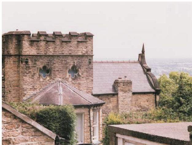
The Oak Tower, at No. 134 Upperthorpe, is a Gothic turret rising to the west of the house for enjoying the south easterly views.
