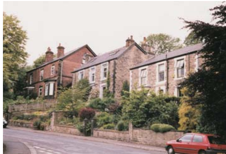
Nos 118 to 124 Upperthorpe, a run of four good houses in original condition
