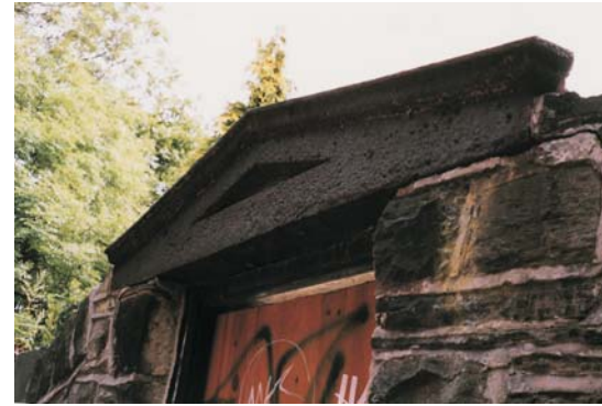
The rear garden wall of 170 Upperthorpe is topped by an unusual triangular pediment made of iron slag.
