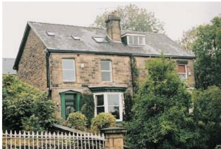
Large rooflights and poorly designed dormers intruded into prominent roof slopes.
