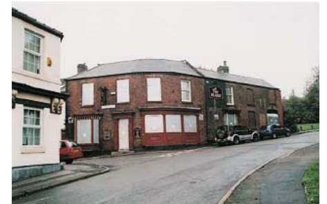
Buildings at risk: the Blake Pub in Daniel Hill Street is boarded up and disused.
