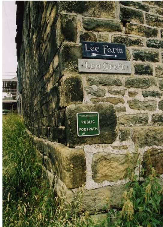
Photograph BHL 8: 1950s cast-iron footpath sign. Note also the plinth formed by the lower three courses of stone of this 17th-century barn.
