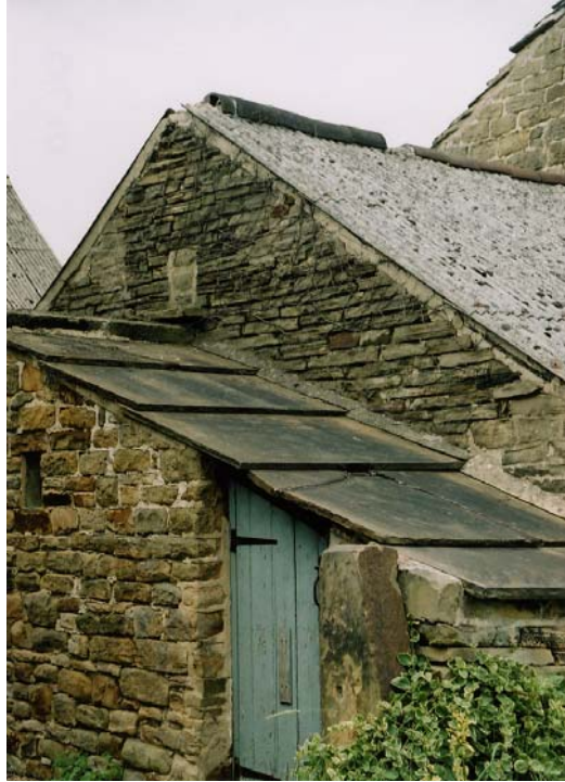
Photograph BHL 10: Pig sty with a roof of massive carboniferous sandstone 'flags'.
