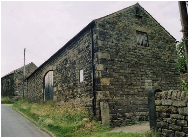
Photograph BHL 6: The barns lining the northern edge of Brightholmlee Road are handsome buildings with an offset plinth up to 1 metre in height, big flush quoin stones, flat-arched cart entrances of cut stone and plank doors. This one also has an owl hole in its gable end and a pitching hole.
