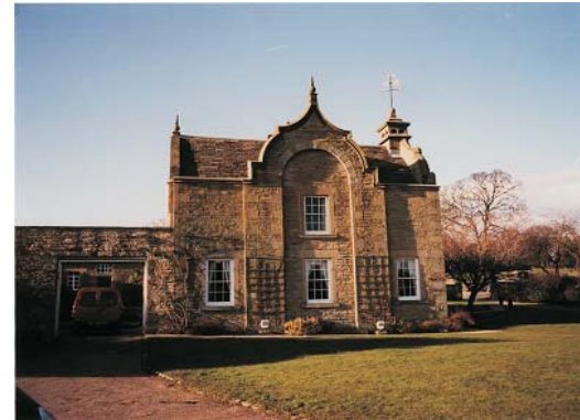
Southern gable of Pegge's Cottage
