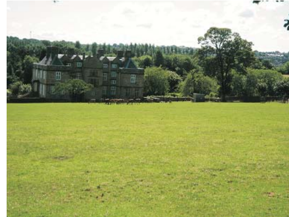
North façade of Beauchief Hall from the woodland walk
