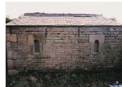
Rear of 'garden shed' in the walled garden
