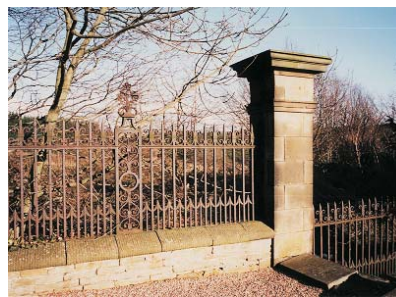
Stone piers and decorative railings around formal garden
