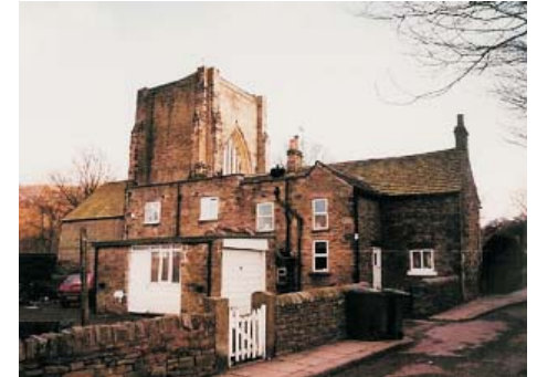
Flat-roofed extension and lean-to garage on rear of Abbey Cottages are out of keeping.
