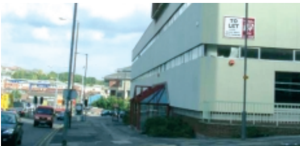
6 – TENTER STREET A VEHICULAR GATEWAY WITH MASSIVE BUILDINGS MARKING ITS CENTRAL BUSINESS DISTRICT CHARACTER
