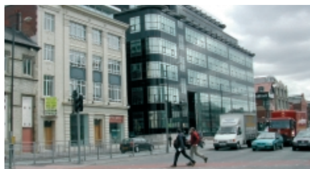
THE EXPRESS NETWORKS BUILDING (MANCHESTER)
