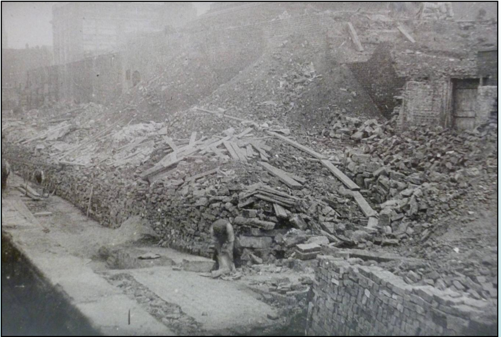
Demolition of Shambles and Chandlers Row for Castlegate, looking east, unknown photographer (Museums Sheffield)
