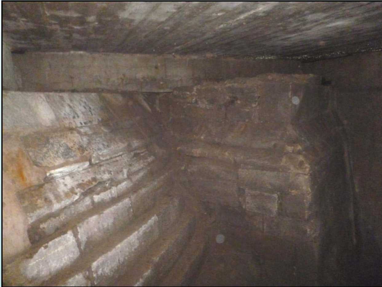
Castle gate structures within chamber, looking north-east, 2013
