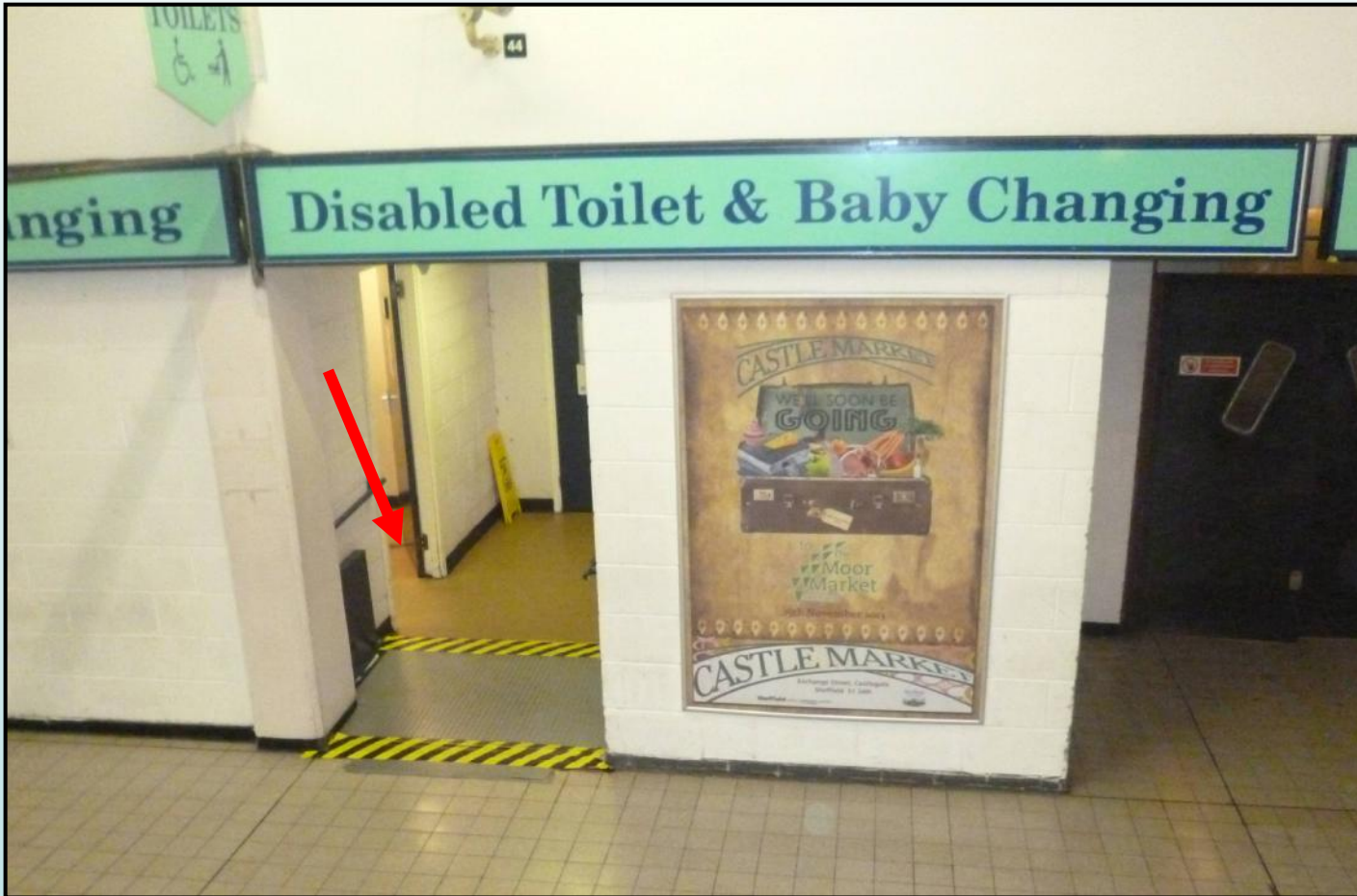
Entrance cover to gate structures chamber, Castle Market, 2013
