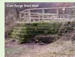
Carr Forge Dam Wall
