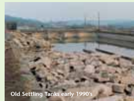
Old Settling Tanks early 1990's
