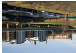
24. Parkway Viaduct carries the Supertram beyond the Park Square roundabout and alongside the Sheffield Parkway link road to the M1. It is a post-tensioned glued segmental reinforced concrete structure 295m long with spans of 55m.
