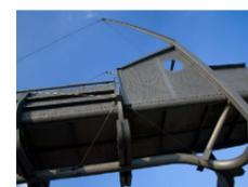
21. The **footbridge** into Ponds Forge Swimming Pool building was required by the client to be "interesting and imaginative". Tensioned cabling is used to stiffen the slender structure.
