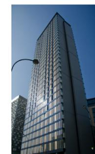
13. **St Paul's Tower**, now the tallest building in Sheffield, is 32 storeys and 101m high plus the basement levels. In-situ reinforced concrete was used for the frame of the building providing a robust core, to which modular cladding was added.
