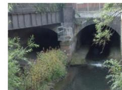
19. The culverts carrying the **River Sheaf** are visible here. It was culverted in the 1860s as the city expanded into the river valley with the development of the railway and market area.
