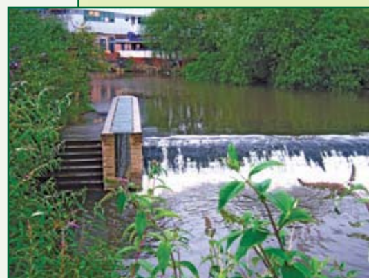
Fish pass in Walk Mill Weir, Effingham Street, Sheffield
