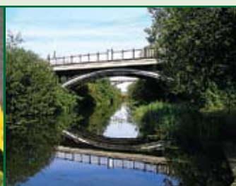
Attercliffe Tram Bridge
