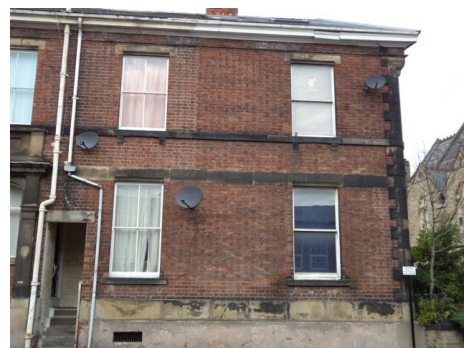
Satellite dishes should be located in unobtrusive positions
