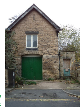
Heritage at risk
