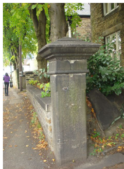
Boundary walls and gateposts are key character features
