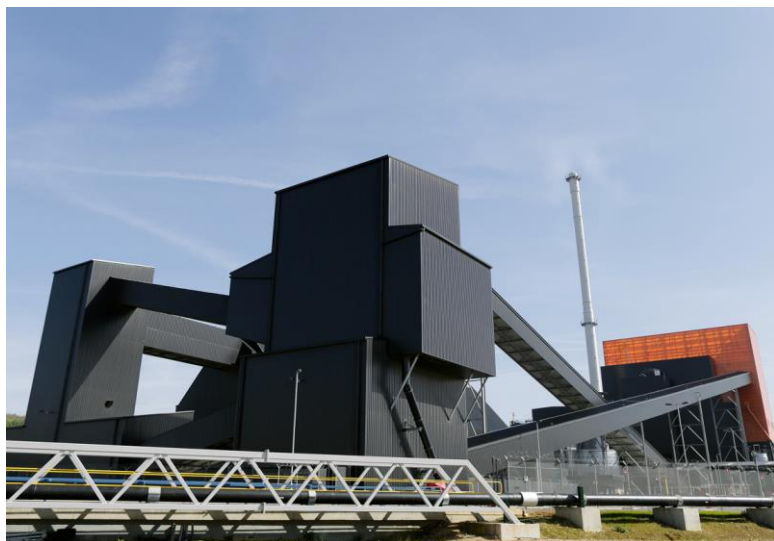
EON, Blackburn Meadows biomass CHP
