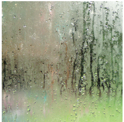
Condensation on a window pane
