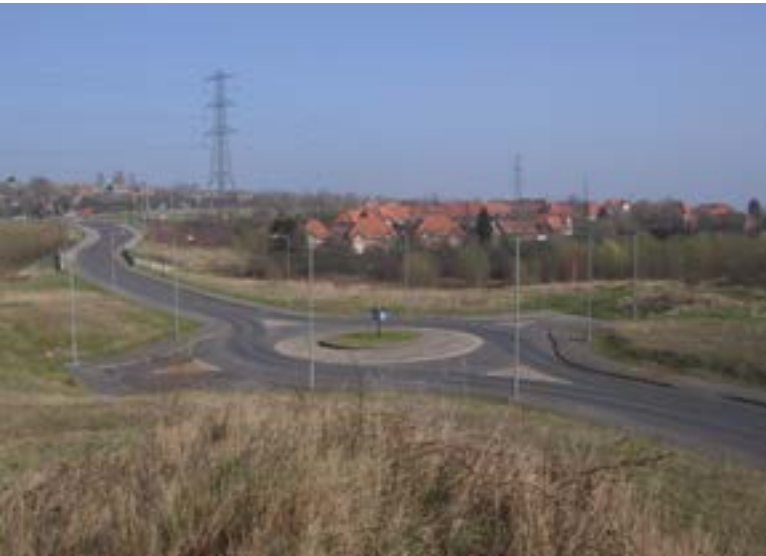
Existing road infrastructure
