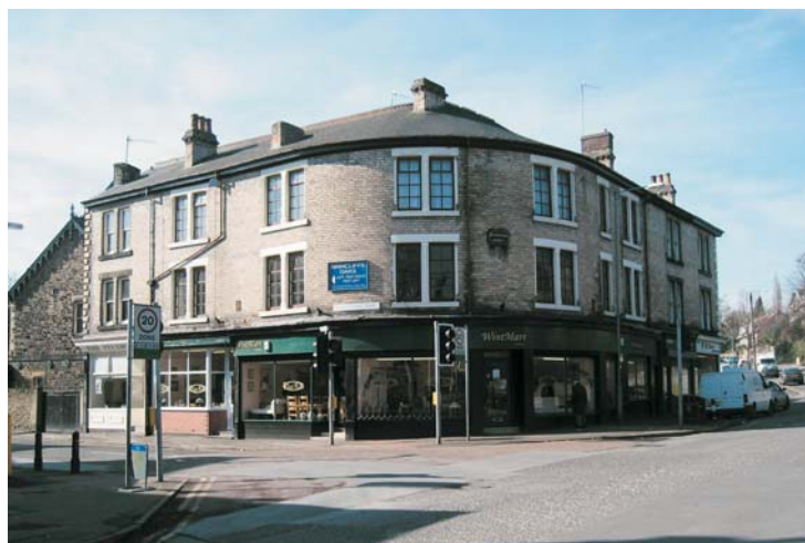
Fig. 27 Nether Edge Shops - an important junction at Nether Edge's only shopping area. The attractively curved corner is a memorable feature.
