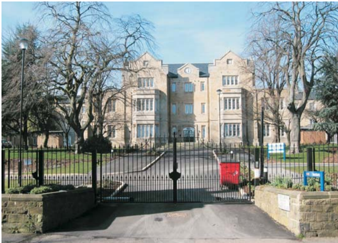
Fig.26 The former Union workhouse and later Nether Edge Hospital, now converted into residential apartments.
