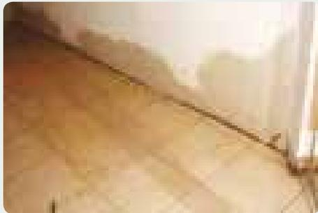
Rising damp shows as a water mark rising up the wall from under the floor.
