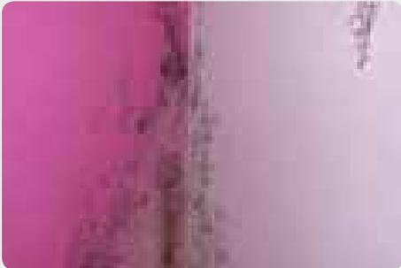
The photo shows a typical pattern of mould affecting the wall in the coldest areas. The shape of the black mould mirrors the temperature of the wall surface.
