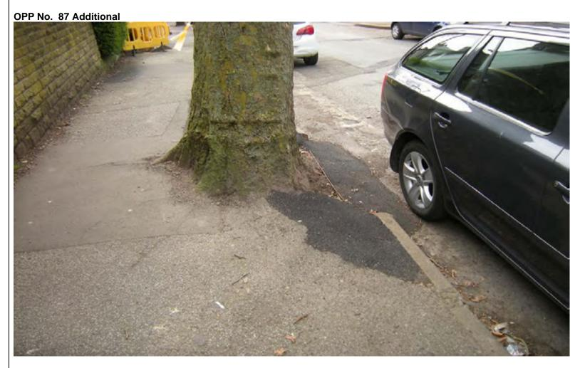
Temporary repair in Bitmac to cover roots into carriageway. Evidence of roots tracing towards property. Previous thin kerb already failed and removed due to roots, unable therefore to replace half kerb.
