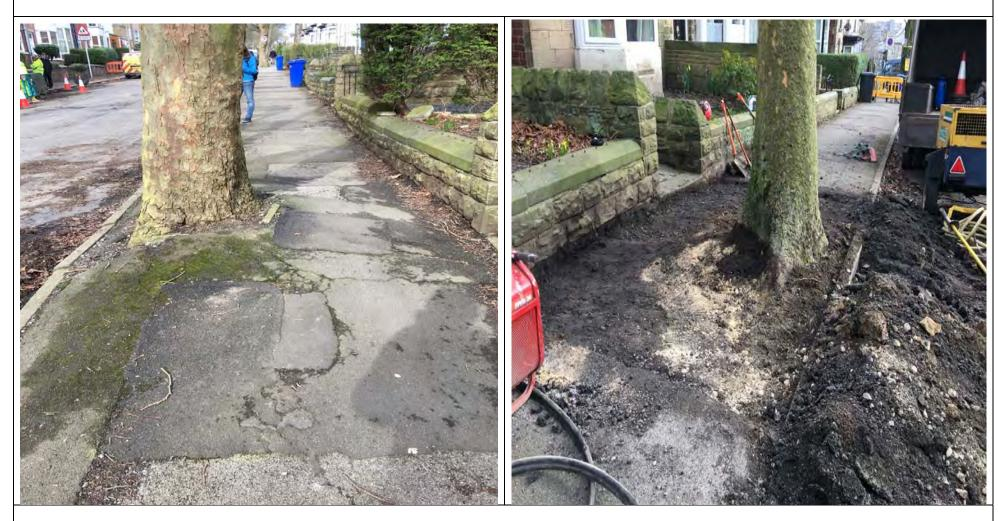
The location of the roots prevents the kerb being correctly aligned and backed up with concrete.
