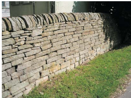
Drystone wall with rounded coping stones, Whirlow Lane
