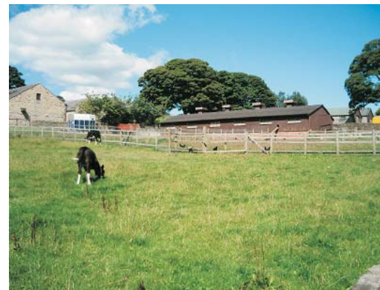
Animal shed from the pedestrian footpath
