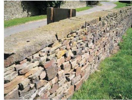
Drystone wall with flat coping stones, Whirlow Lane
