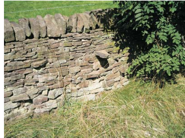
Stone wall beside verge, Whirlow Lane
