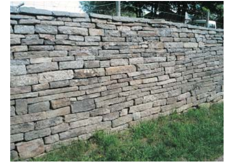
Stone retaining wall, Whirlow Lane
