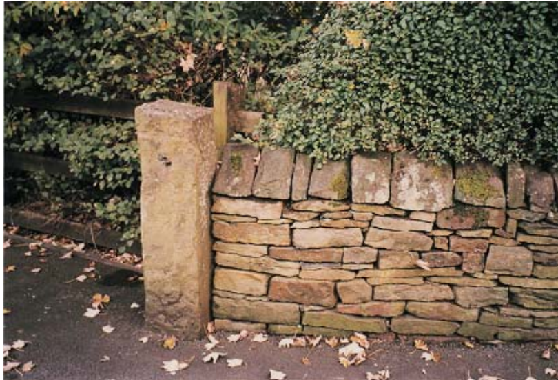
Characteristic stone wall with triangular coping
