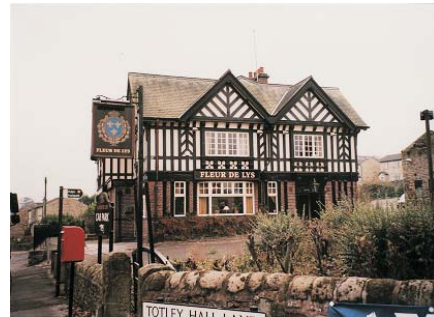
North façade of the Fleur de Lys public house
