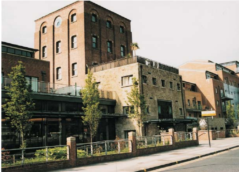
The brick brewery tower, built in 1874, of the Sheaf Brewery, Ecclesall Road, is now part of a large residential development of 2002 by Finnegan Design and Build.
