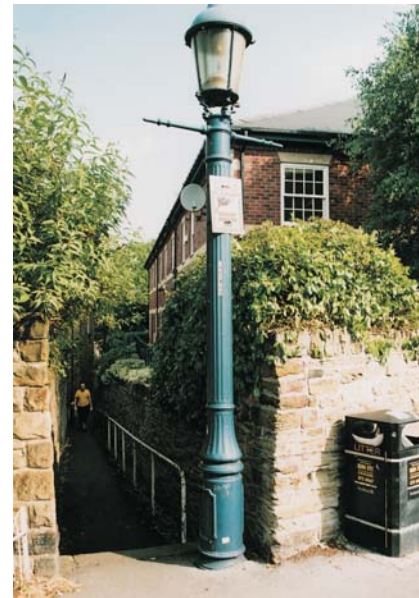
Sewer Gas Lamp, Cemetery Road and Frog Walk junction, Grade II, late 19th-century and still in working order.
