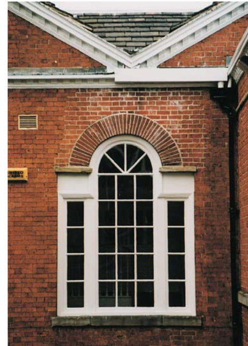
Westbrook House, Sharrow Vale Road, Grade II, 1795: the rear elevation has a Venetian stair window.
