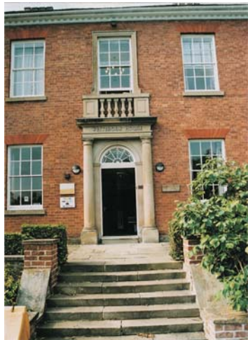
Westbrook House, now converted to offices, is a Grade II listed building in the Conservation area
