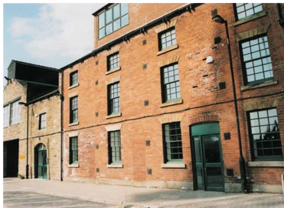
Sheaf Brewery is entirely accessible, with paths linking Pomona Street and Harrow Street that pass through the complex and allow sight of the historic buildings that survive.
