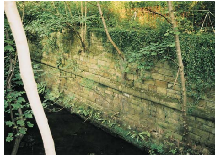
Listed retaining walls to the Porter Brook.
