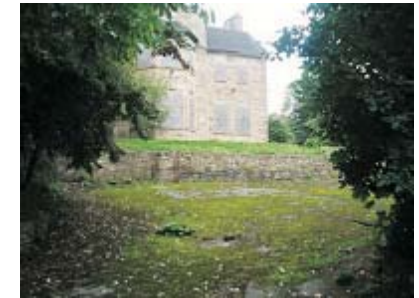
No. 84 Norfolk Road is vacant and boarded up.
