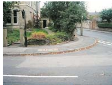
A boundary wall has collapsed at no. 71 Norfolk Road.
