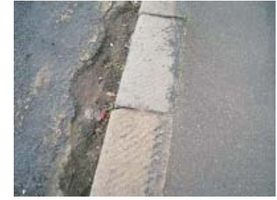
Stone kerbs typical of the conservation area.
