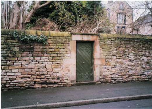
Door in high stone wall, Claywood Road
