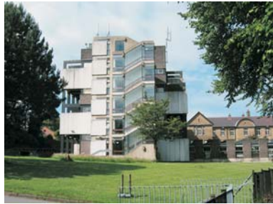
(a) Sheffield Hallam University - ugly modern extension to attractive Edwardian former school.
