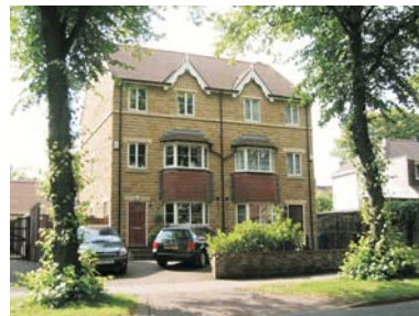
(j) The proportion of floor heights, bay windows and dormers are at odds with the local character despite attempts to copy the local style.
