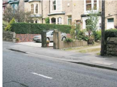
(f) Creation of vehicular accesses can break the continuity of boundary walls and isolate gate posts.
