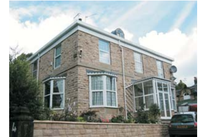
(h) The replacement of timber windows, doors, porches, soffits and barge boards with UPVC affects the traditional character & appearance of historic buildings.
