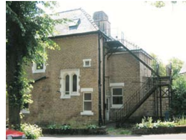
(c) Flat conversions of large houses often create the need for intrusive fire escapes.
