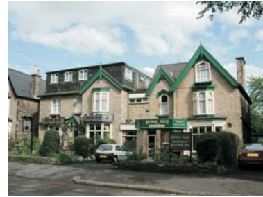
(g) Roof dormers which damage traditional roof forms.
