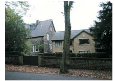
(d) Modern infill with different scale, roof pitches and window proportions to neighbouring Victorian Villas. The close proximity of the new house also impinges on the setting of the villa.
