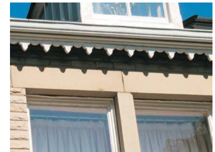
(l) Stone sills and lintels.
