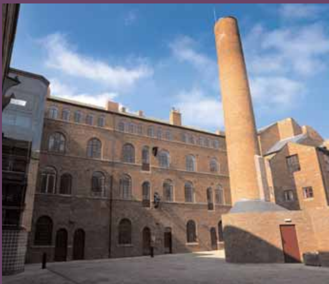
Figure 16: Internal courtyard after works were completed
