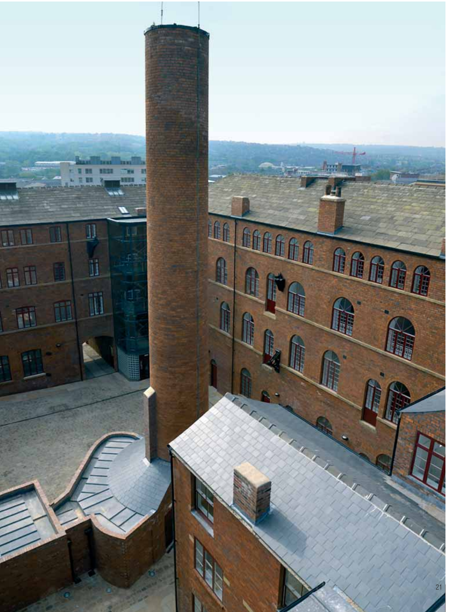
Figure 14: Butcher Works: The impressive chimney and internal courtyard after restoration
