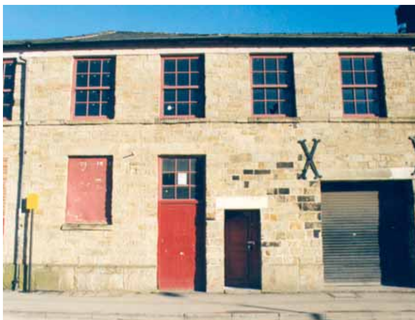
Figure 12: Scotia Works before works supported by the THI commenced
