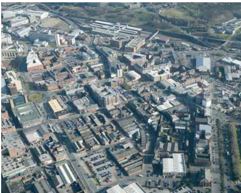
Figure 1: Aerial photograph of CIQ area and historic photographs of Arundel Street
