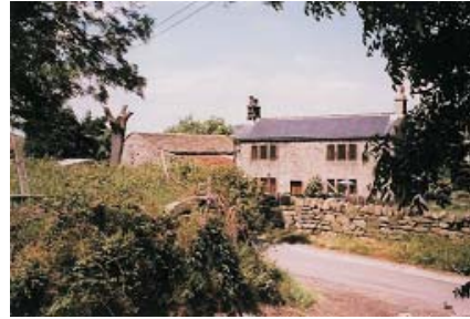
Replacement doors and windows, and cut down trees.
