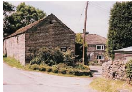
Replacement doors and windows, and insensitively sited sheds.
