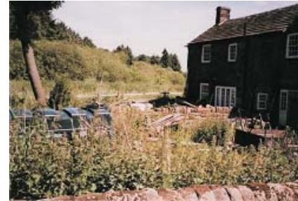
Ongoing building works and prominently sited oil tank.
