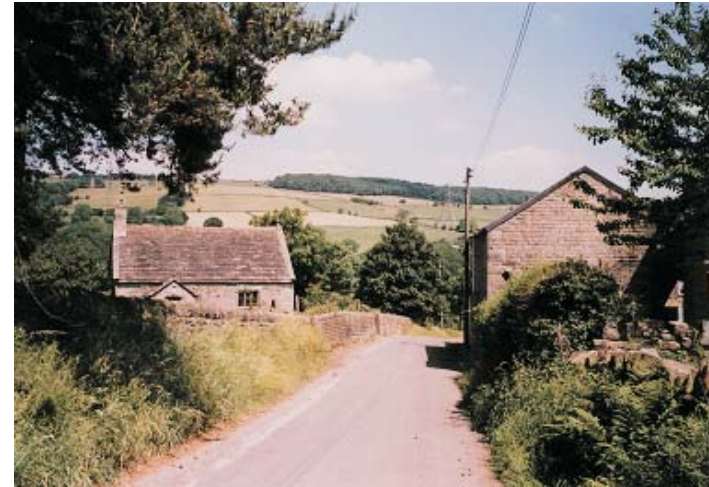
Cart sheds help to define the edge of the sunken lane between Stoneycroft House and Midhope Hall Farm.
