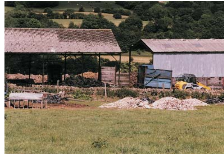
Builder's rubble and farm waste detract from the appearance of the conservation area.
