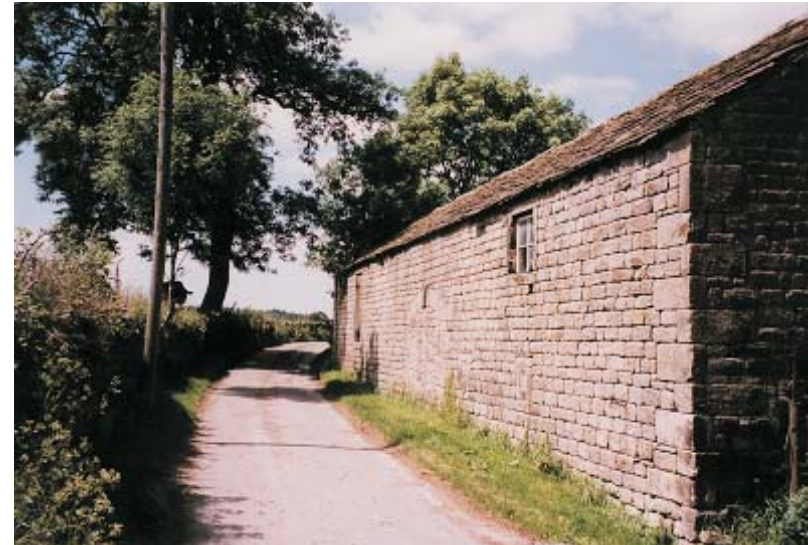
19th-century barn with blocked cart shed entrance beyond Stoneycroft House.
