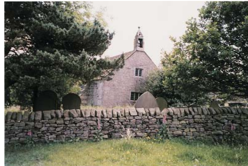
The gritstone walls surrounding the churchyard have a mix of triangular and semicircular coping stones.
