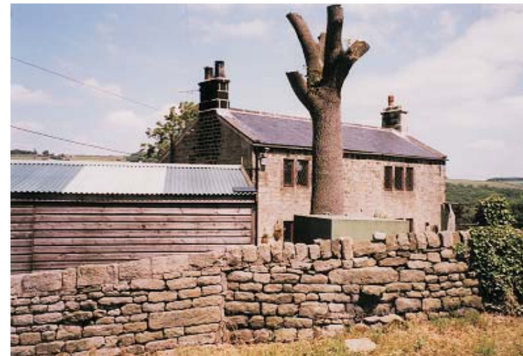
This modernised farmhouse has lost much of its character through the use of non traditional window materials and the prominent siting of the shed and oil tank, as well as the severe lopping of the tree.
