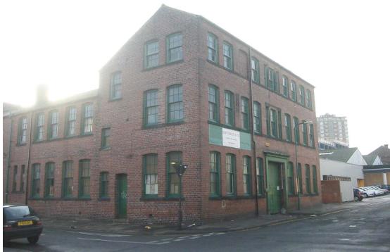
78. S. Murray and Co. (1) on Boston Street (listed Grade II) - an almost text-book example of a metal trades factory.
