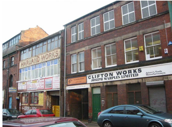
85. Harland Works (7) and Clifton Works (8), adjacent to Stag Works - both make key contributions to John Street.
