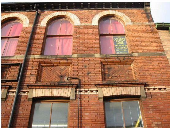
100. Brickwork detailing to Randall Street elevation of Portland Works.
