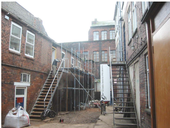
86. Courtyard to rear of Harland Works (7) and Clifton Works (8) - the rear face of Portland Works (10) can be seen in the background.
