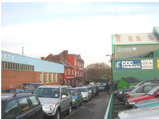
88. Looking east along John Street - more recent development is now visible in the foreground.
