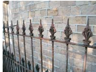
A short length of historic iron railing at Hackenthorpe Hall.
