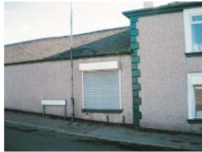
Roller shutters deaden the front of a building.
