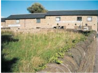
Old stone boundary wall with half-round stone coping.
