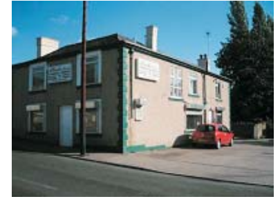
A historic stone building altered by the application of a modern render.
