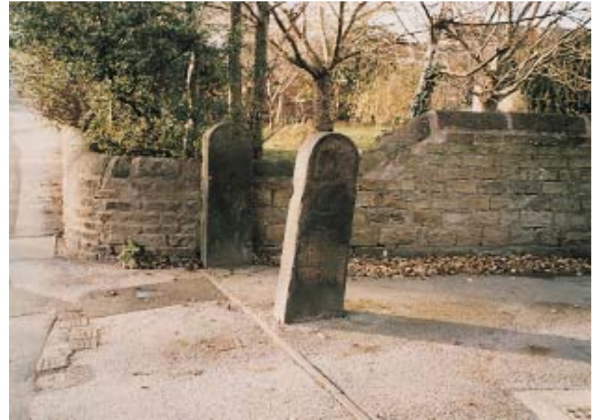
Stone pillars at entrance to Brookhouse Court
