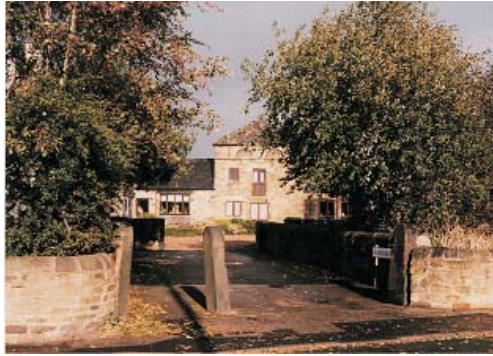
Entrance to Brookhouse Court
