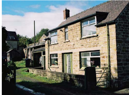
Replacement of traditional timber windows and doors.
