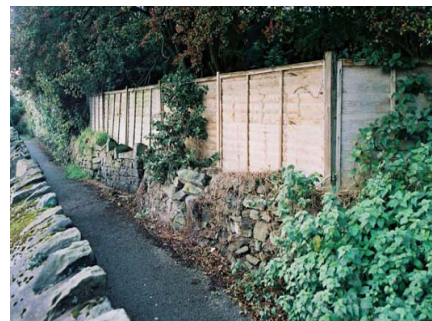
Uncharacteristic timber fencing.
