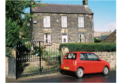
Front elevation marred by drainage pipes, wiring, burglar alarms, exterior lighting and satellite dishes.
