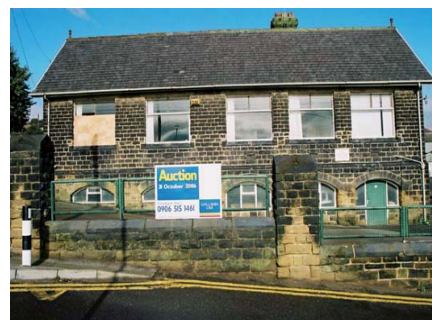
The former Grenoside Infant School on Norfolk Hill is vacant but has outline planning permission for residential conversion.
