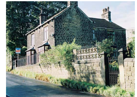
Replacement windows and garden walls built of patterned breeze block.
