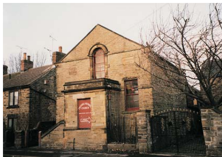
Methodist Chapel, Greenhill Main Road
