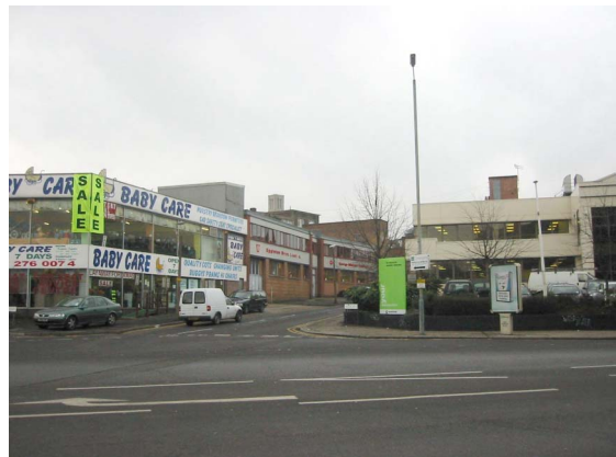
10. Inappropriate development along Allen Street - view looking south-west.
