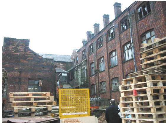
40. Rear yard of Don Cutlery Works accessed via Shepherd Street.
