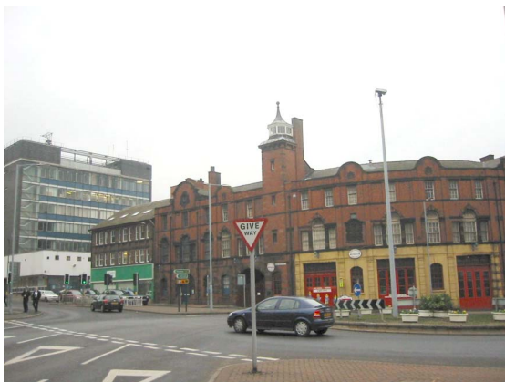
5. The Fire Station Museum (12) on the corner of Westbar Green and Gibraltar Street (listed Grade II). The Police Station can be seen background left.
