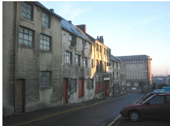
18. The John Watts Cutlery Works (1) on Lambert Street (listed Grade II).
