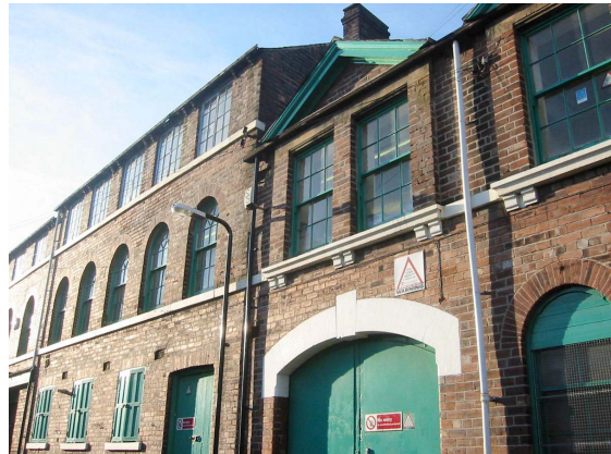
34. Kutrite Works on Snow Lane (4) (listed Grade II) - note the different treatments of ground, first and second storey windows.
