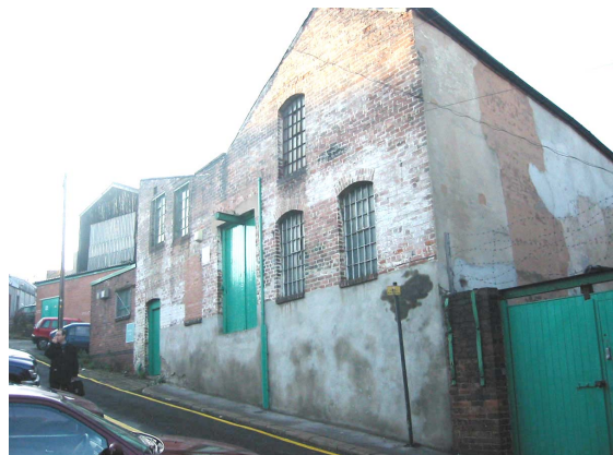
36. Adjacent to Kutrite Works on Snow Lane are these plain brick buildings with cast iron small-pane casement windows.
