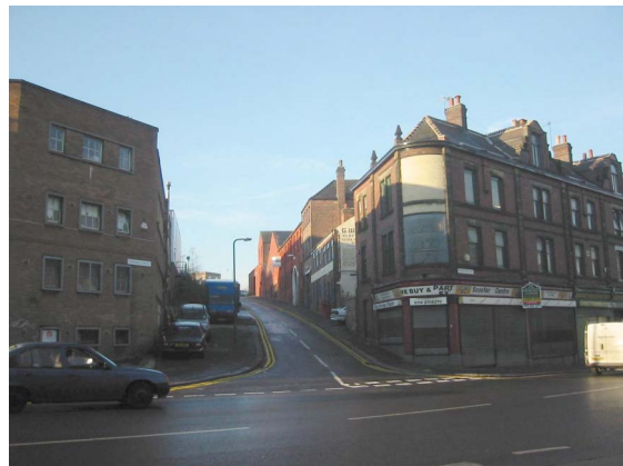
22. Looking west up and along Furnace Hill - towards GW Potts Works (3) and Hope Works (2).
