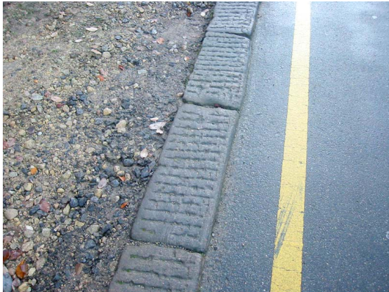
31. Sandstone kerbs with tooled grooves to provide grip on steep inclines.
