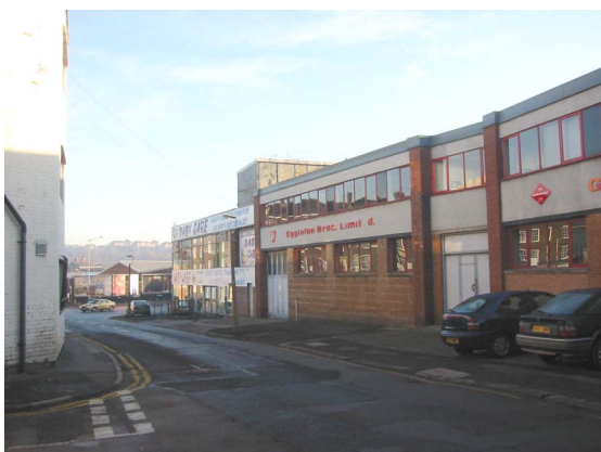
11. Further view of later buildings along Allen Street - looking north-east.
