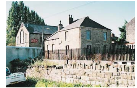
Buildings a risk: the Wesleyan Chapel and Sunday School in the High Street.
