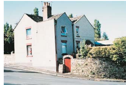
Large extensions that do not match the original building in terms of material, colour or scale.
