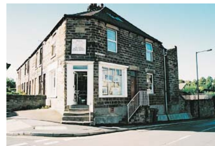
A good historic shopfront with original door and stone steps.
