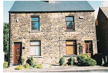
Traditional timber windows and doors replaced with leaded diamond sealed units.
