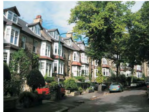
Rutland Park (west side)
