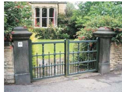
Typical stone gate piers and stone boundary wall.
