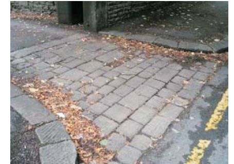
An area of stone setts and kerbs at the entrance to a large dwelling.
