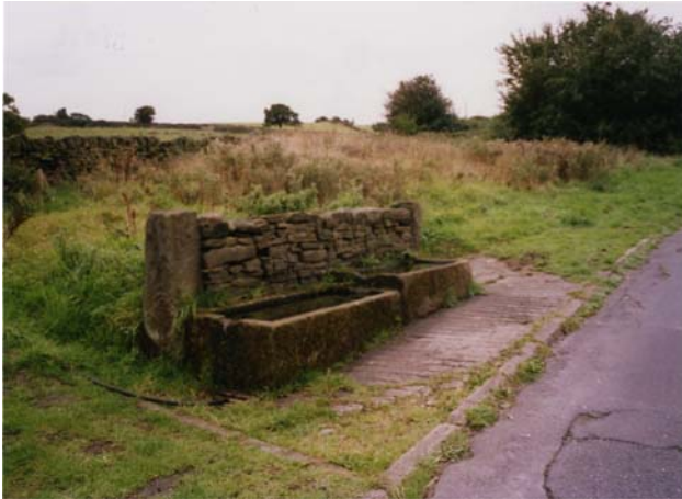
Replacement of the concrete surround with more traditional materials, such as cobbles, would enhance the setting of these two large sandstone troughs.
