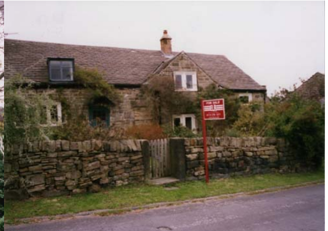
Modern alterations to a historic building.
