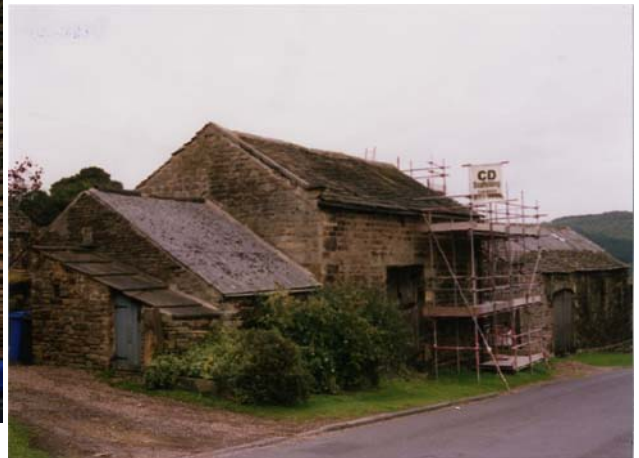
Scaffolding stabilising a barn wall at Old Hall Farm
