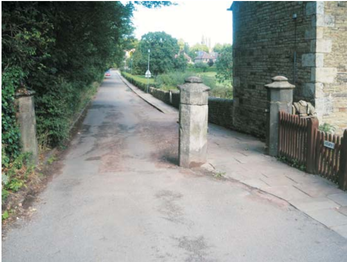
Three stone piers at north end of 'causeway' (Beauchief Abbey Lane)
