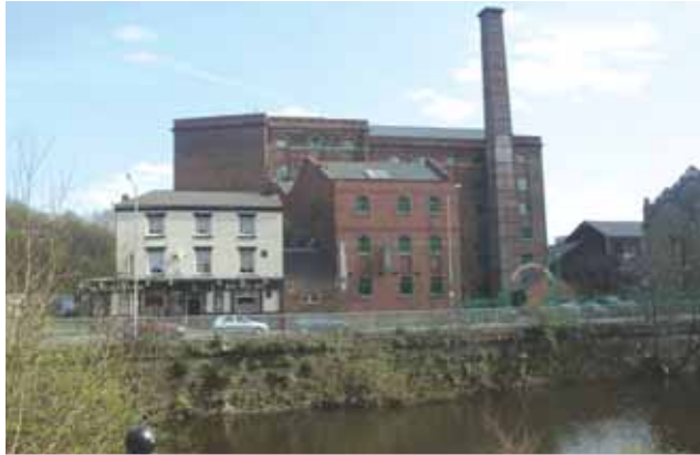
AIZLEWOODS MILL, NURSERY STREET
